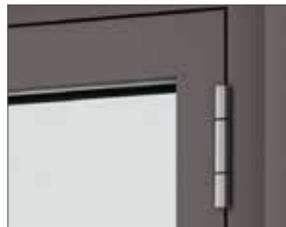
**Barrel hinge** with or without security bolt. Natural anodised surface finish.
