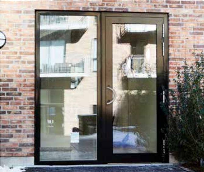
1-LEAF DOOR WITH 160MM GLAZING BAR, PANIC BAR AND BARREL HINGES IN A VELFAC 200 SCREEN
