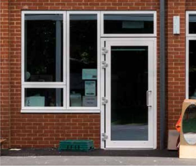
2-LEAF DOOR WITH ANTI-FINGER TRAP HINGES, AND FULL HEIGHT PULL HANDLES
