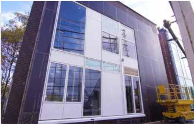
VELFAC offers a CWCT accredited solution. The 62m<sup>2</sup> large window wall made with 8 complete window units, 20 individual sashes, 6 large opening functions and 5 panel solutions is tested for air permeability, water tightness and wind resistance.
