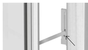
> **The lockable restrictor** limits the opening of the sash to 1.5-10cm. It is possible to disengage the restrictor by turning the lock through 90° with a 5mm hexagon key. Now the restrictor arm may be pushed out of the gliding rail. The lock must always be re-engaged after use. The gliding rails should frequently be cleaned from dirt.
